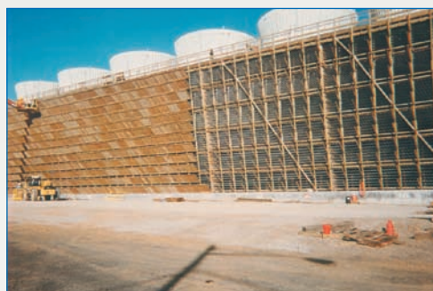
Replacing louvers
